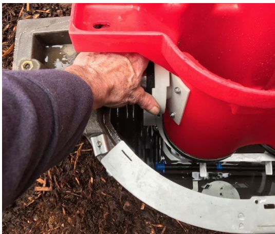
STEP 6: Rotate the fastening nut left or right 90 degrees to free the collar from the filter carriage and pull back on the accordion tube.
