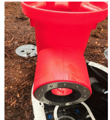
STEP 7: Pull back of the filter carriage to clear the metal wash assembly then lift the filter carriage out.
